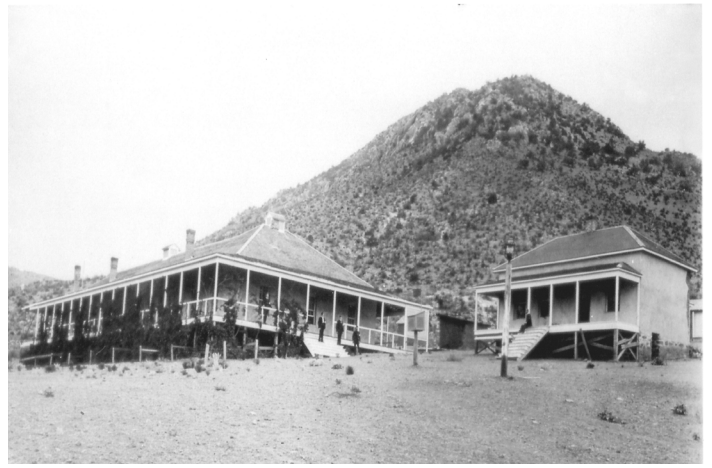
The post hospital at the second Fort Bowie.
